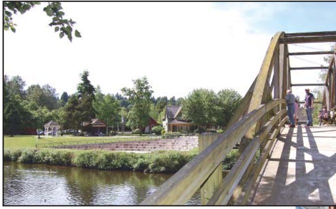
Destination Bothell: bridge connecting the Sammamish River Trail to Bothell Landing
